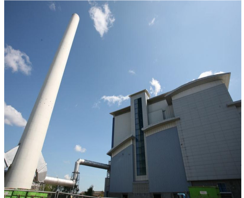
Flue Gas Treatment
